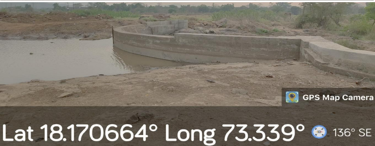
Photos 2: Bunds (Bandara's) constructed on river near Nursery in University Campus
