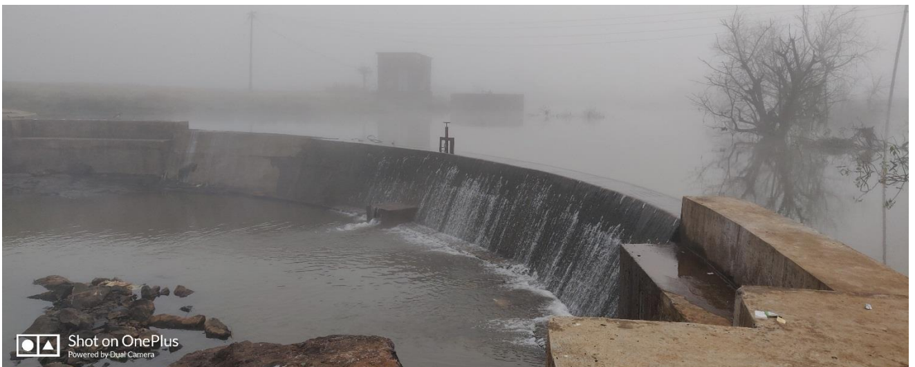
Photo 4↑, 5↓: Concrete Barrage No.1 in arch shape to take advantage of V shaped rocky gorge
