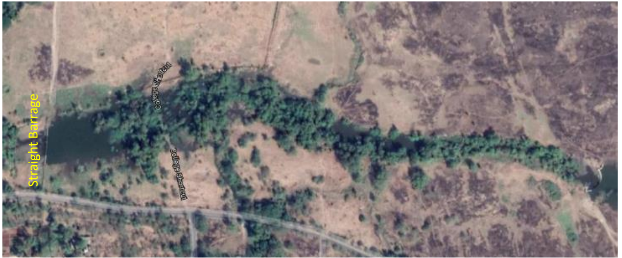
Photo 9: Reservoir created upstream of Barrage No. 2
