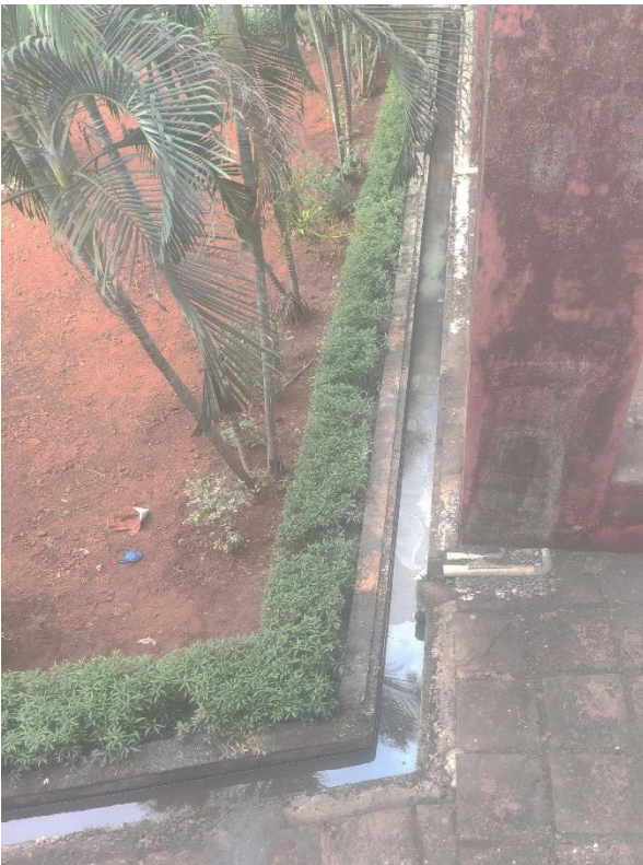
Photos 1 to 4: Rain water collection system at Main Building of University
