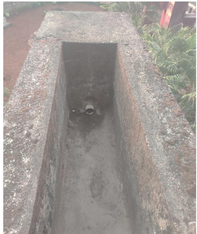
Photos 1 to 4: Rain water collection system at Main Building of University
