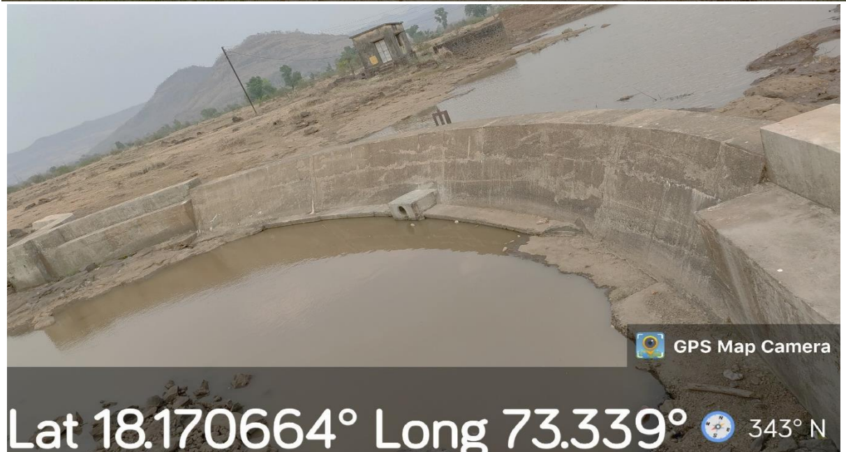
Photos 6 to 7: Bunds (Bandara's) constructed on river near Nursery in University Campus
