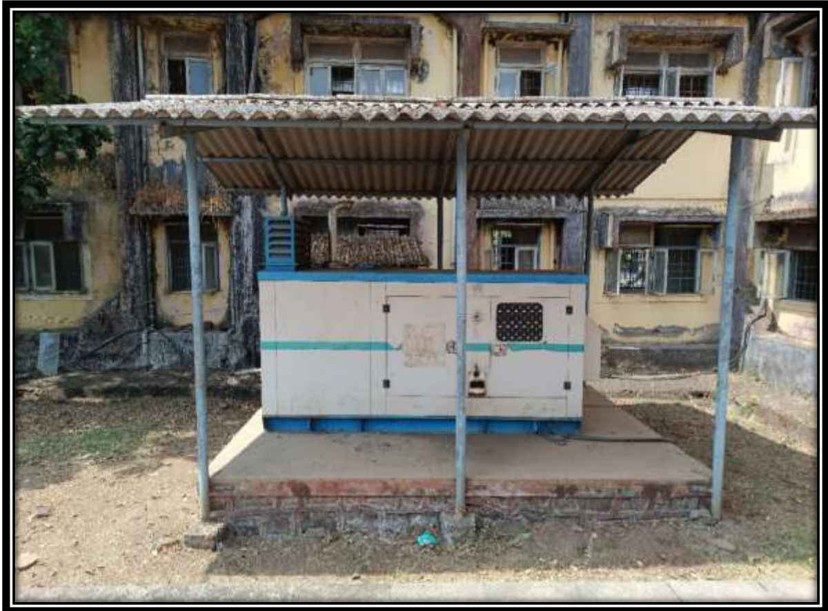
DG Set used for Emergency power supply
